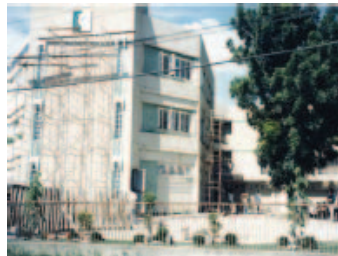
1996. Construction of new building
